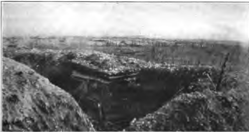
BILLEMONT TRENCHES, NEAR FORGES WOOD
