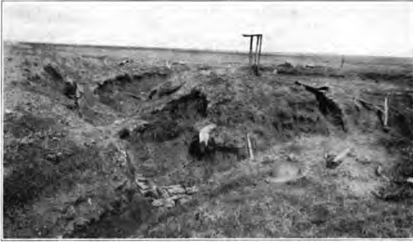
CAPTURED GERMAN TRENCHES NORTH OF BRAY-CORBIE ROAD
