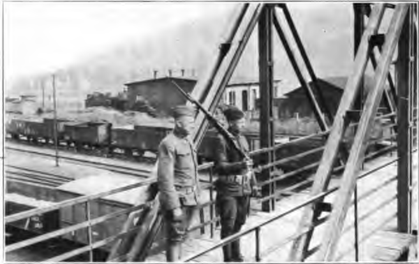
GUARDING LINES OF COMMUNICATION AT WASSERBILLIG, LUX. OBERBILLIG, GERMANY, ACROSS RIVER
