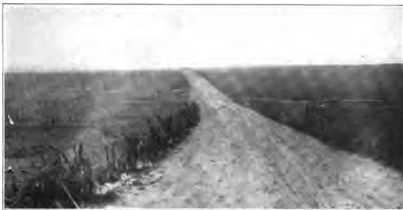
LOOKING WEST TOWARD DOUBLE TELEGRAPH POLE ON BRAY-CORBIE ROAD
